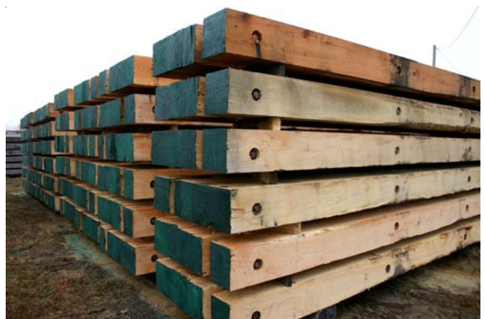
Timber crane mats ready for placement
